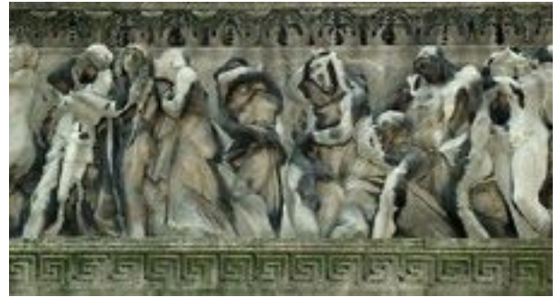
Statues damaged by acid rain
